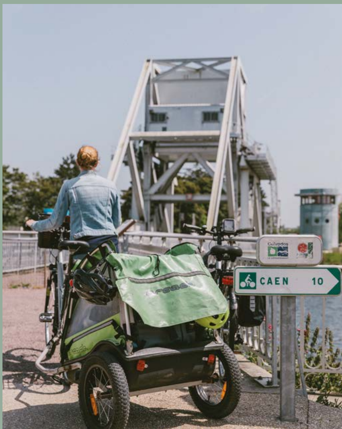
Pegasus Bridge - Bénouville
